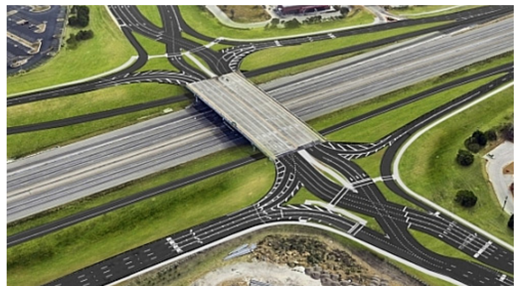
The diverging diamond intersection will temporarily switch the lanes when drivers cross I-35 on Parmer Lane, so drivers will be on the left side of the road. (Courtesy Texas Department of Transportation)
